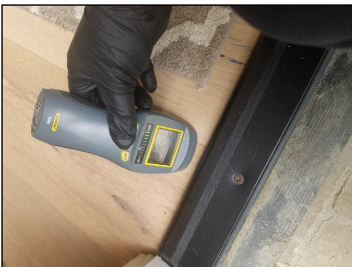
23. Damaged, cracked or loose
