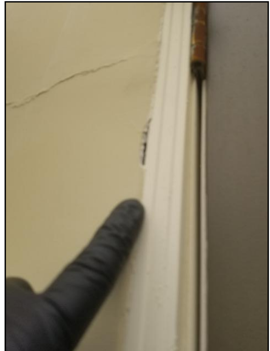
12. Minor cracks
