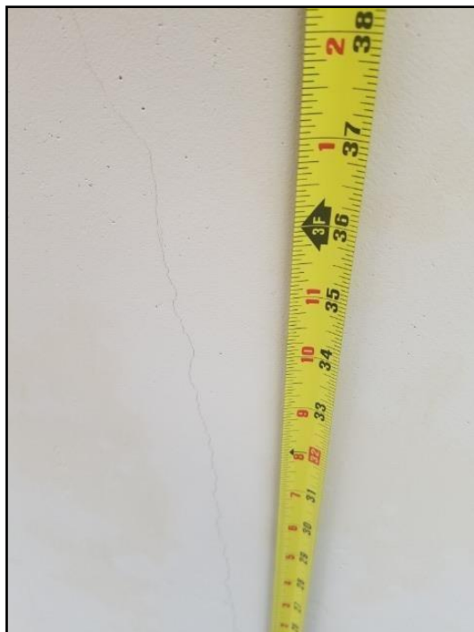
51. Minor cracks
