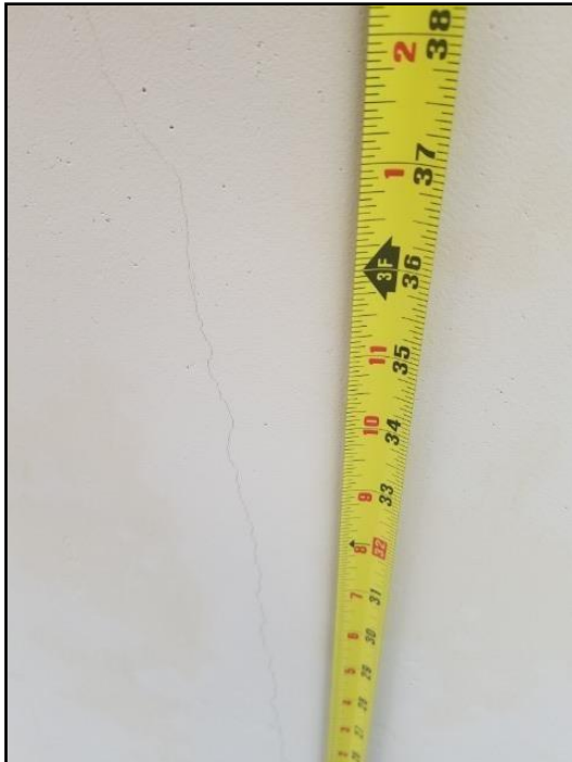
11. Minor cracks
