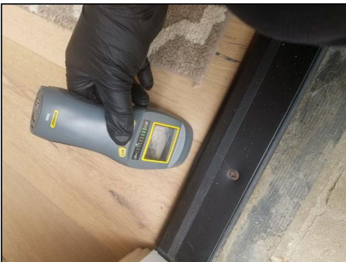
63. Damaged, cracked or loose
